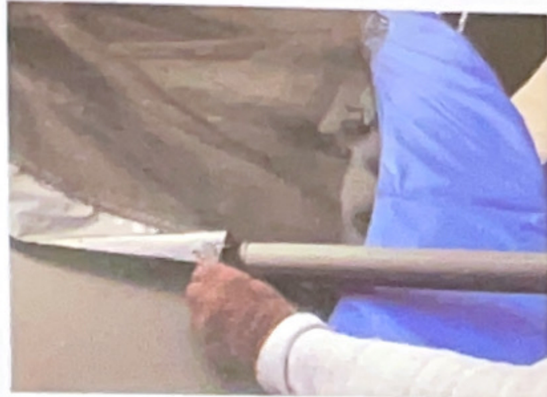
13. Put up safety pole into sleeve
