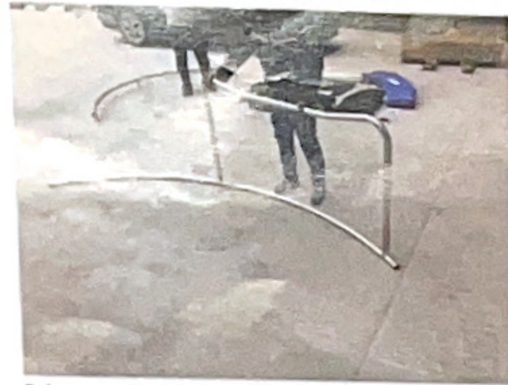
2. Insert the U-leg, this is an assembly then do it one by one
