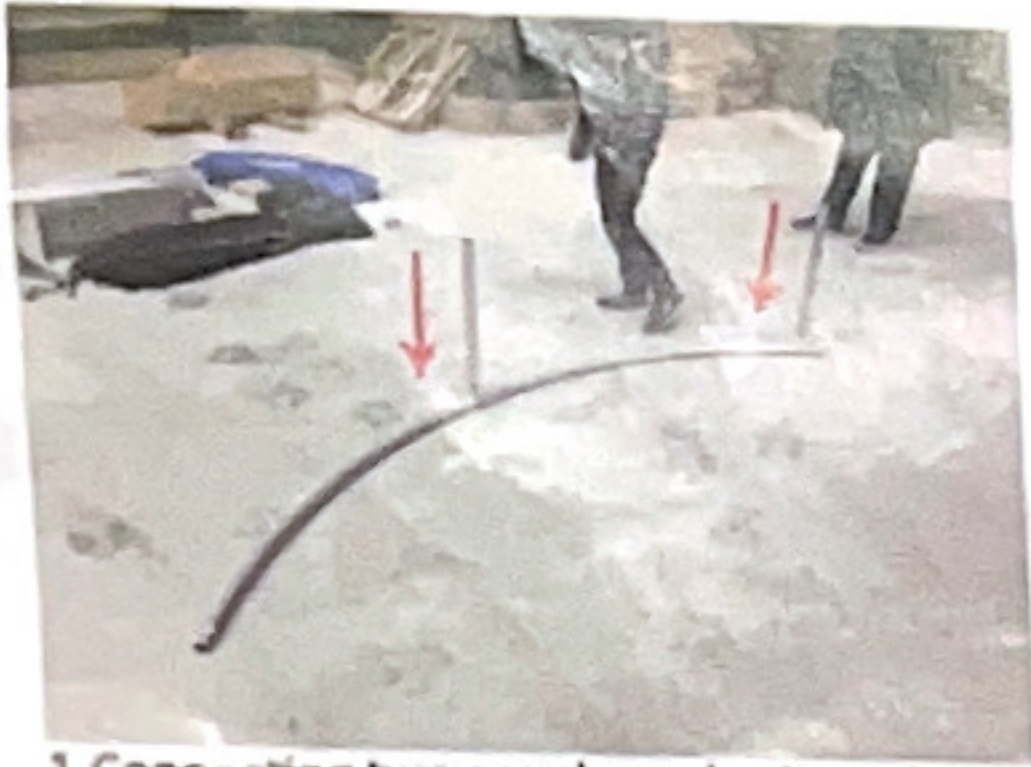
1. Connecting two arc-shaped tubes, then insert connecting tube
